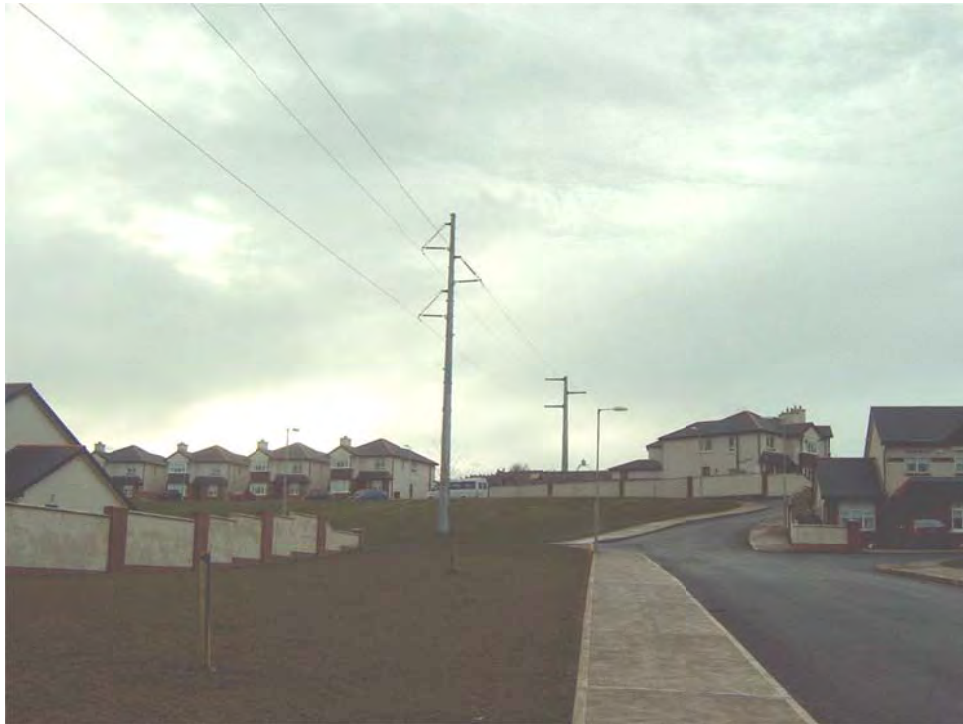
Photo 2: 110 kV Monopole Overhead Line in Cork
